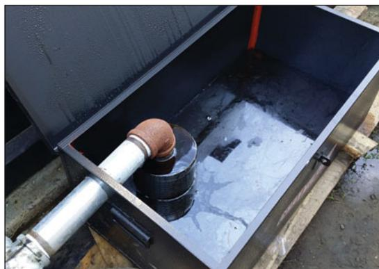
**Figure 3: The tank for collecting condensate.**
